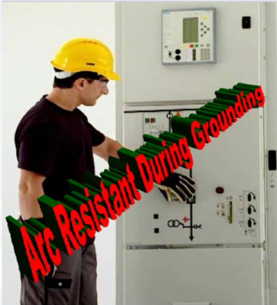
Grounding Using 3-Position Switch Arc Resistant during Grounding
