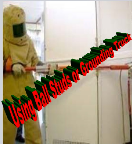
Traditional Way of Grounding NOT Arc Resistant during Grounding
